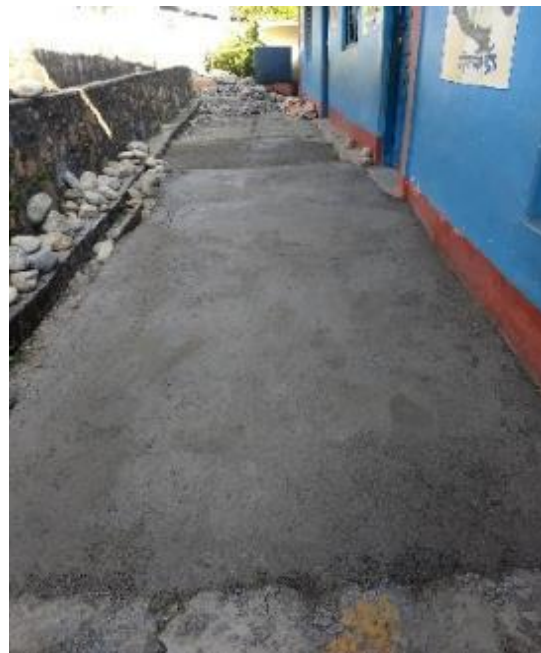
Construction work at Schools (Annapurna)
